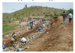
Construction of soil and water conservation structures
